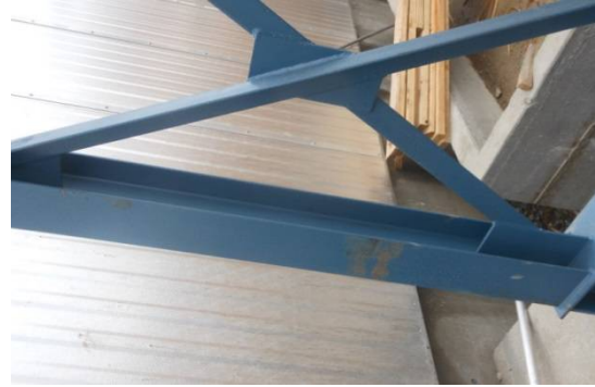
Bent X-Brace/welded
